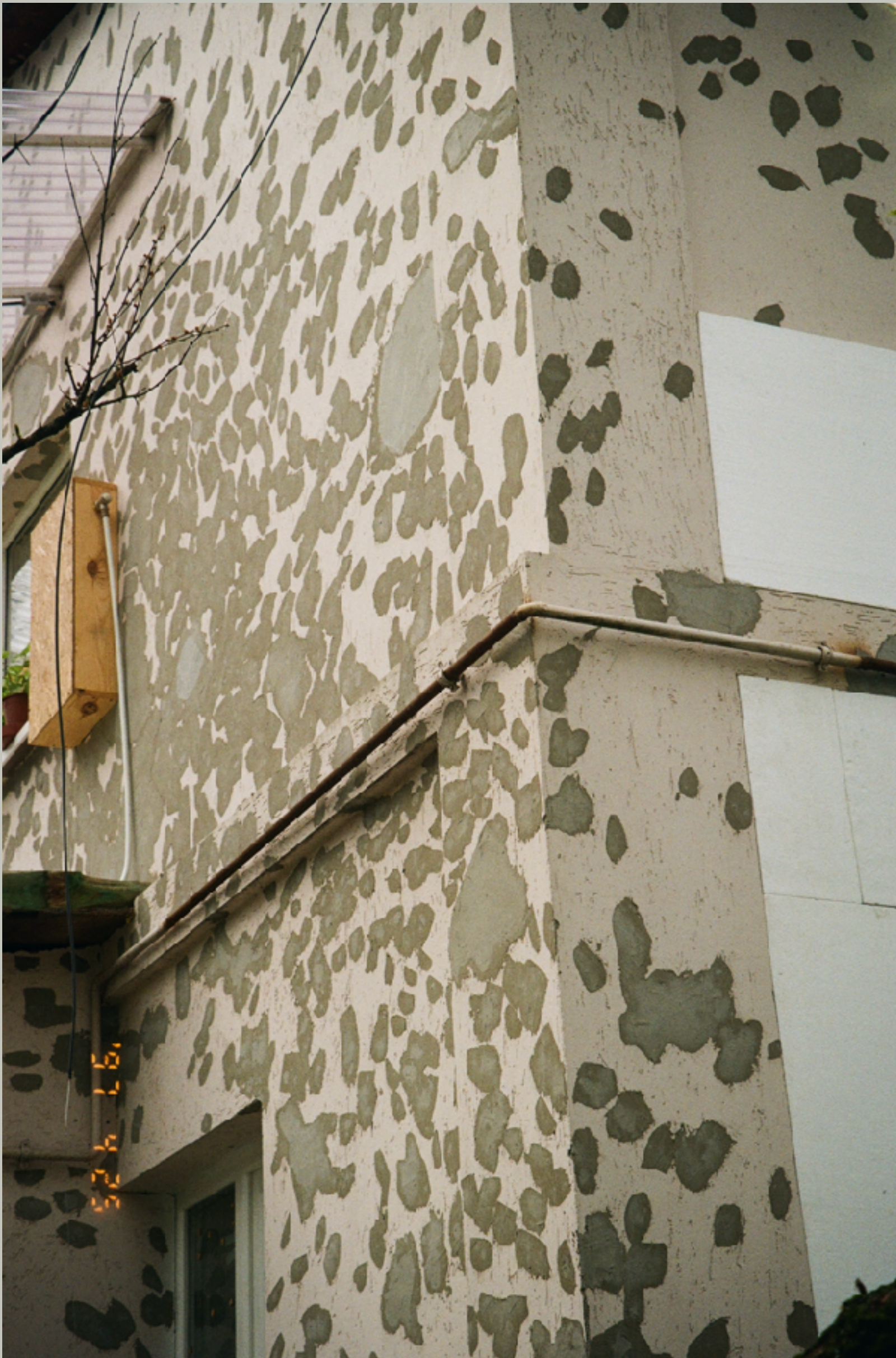
The house repaired after the shelling. Bucha, Ukraine. Spring, 2023
